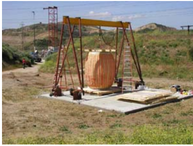
Figure 18. Airlock Supported on A Frame
